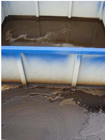
Fig. 9: Oil separator.
